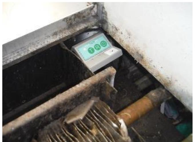
GT sensor mounted on bracket
